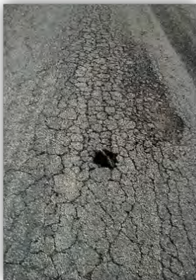
Alligator Cracking
