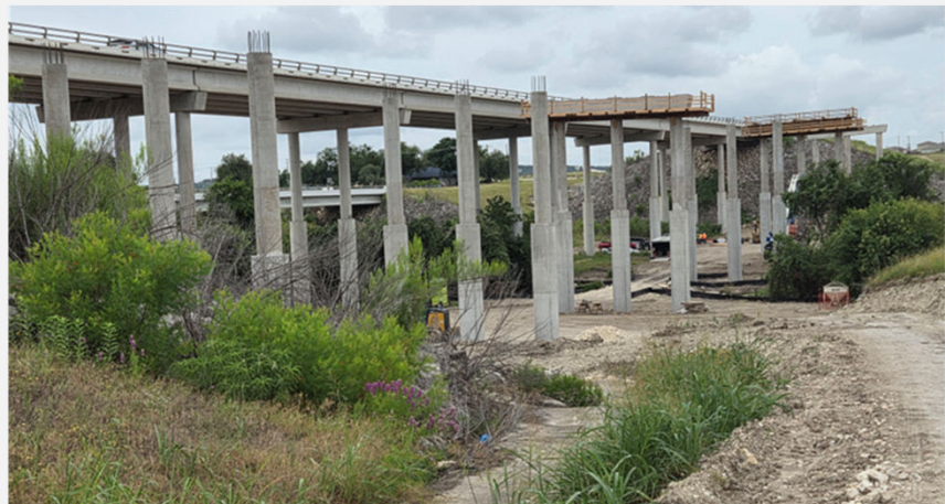
Clear Creek Bridge
