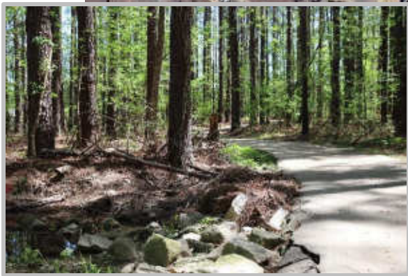
Walking trail is eroding and needs to be repaired
