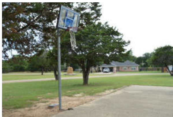
Routine maintenance includes such things as clean up, repairs, and replacement of broken or damaged park elements.
